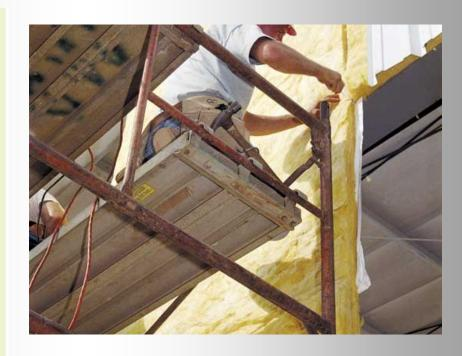
MBI products range from 3 3/8" to 9 1/4" thickness of NAIMA 202-96 Certified R Metal building insulation laminated to a variety of vapor retarders.
