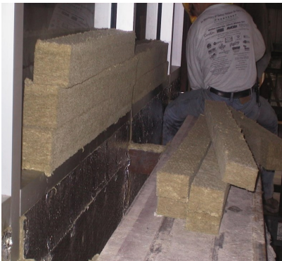
Precut Insulation & Safing
