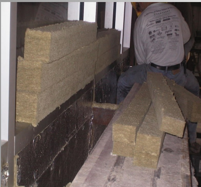
Precut Insulation & Safing
