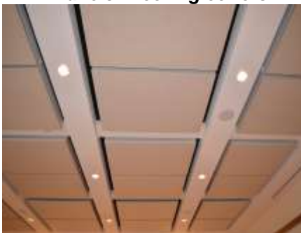
Panels in ceiling coffers
