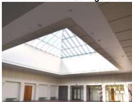
Atrium Wall and Ceiling Panels
