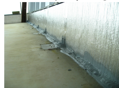
Curtain wall and safing insulation Installed with firestop coating
