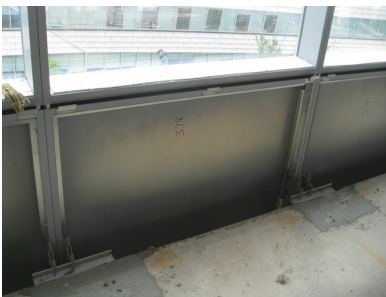
Curtain wall framing
