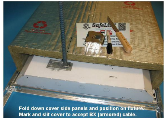
Main Panel Installation (Step 2)
