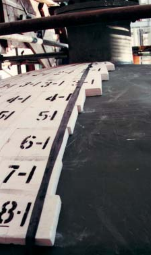
Pamrod HATS installed around a center nozzle.
