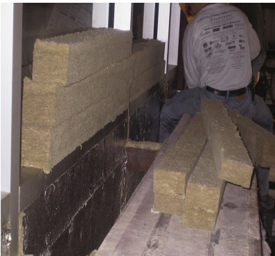
Precut Insulation & Safing
